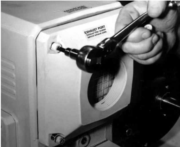
Figure 4 - Removing Exhaust Housing
